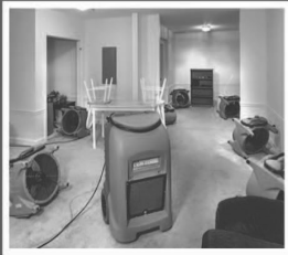
Structural Drying
